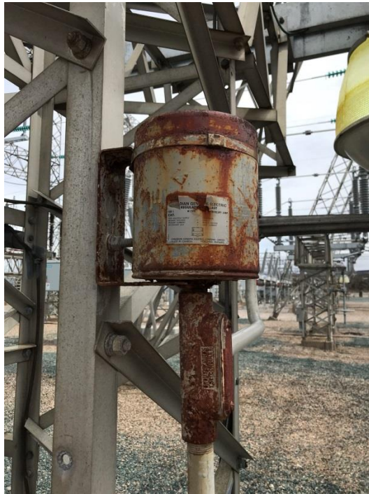
Figure 13: Corroded Ballast Requiring Replacement
