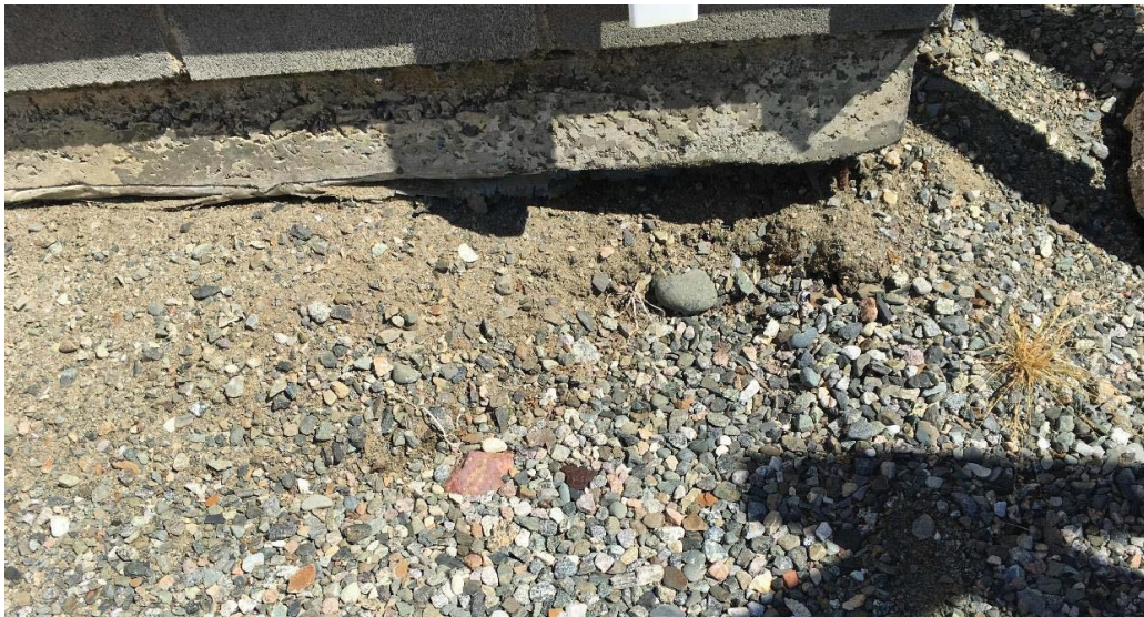
Figure 13: Undermining of Concrete Foundations
