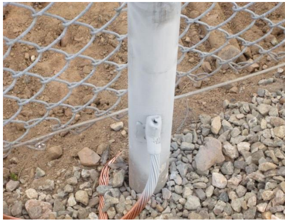
Figure 7: Typical Grounding Connection on Terminal Station Fence
