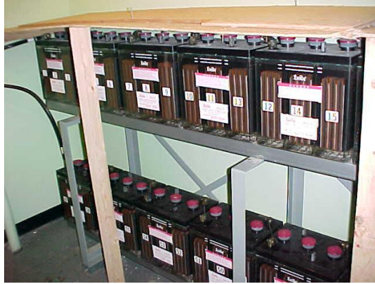
Figure 11: 125 Vdc Terminal Station Battery Bank
