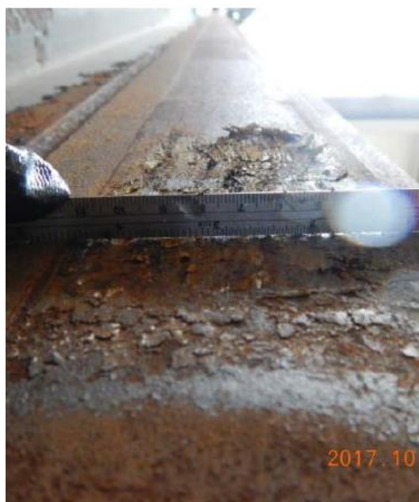
Figure 9: Rubbing Marks on Embedded Parts - Burnt Dam
