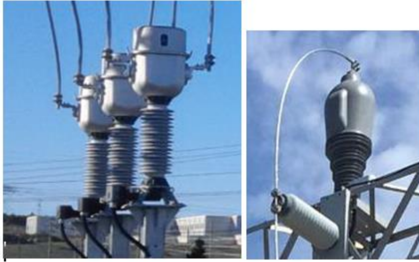
Figure 1: 69 kV CT (Left) and PT (Right)
