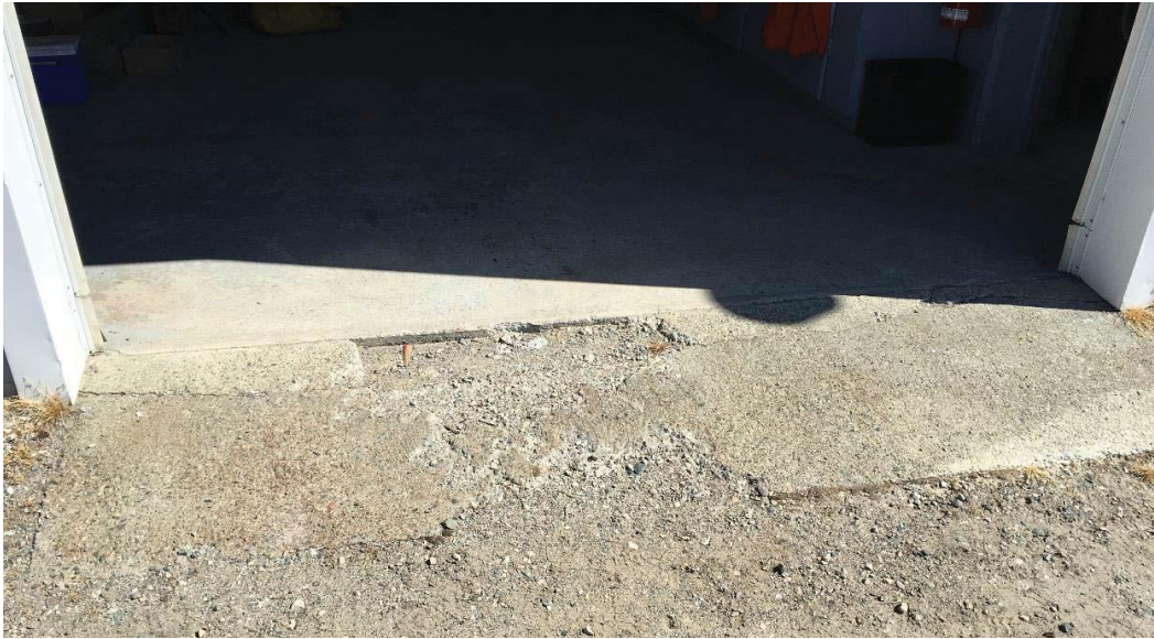
Figure 12: Deteriorated Concrete Ramps
