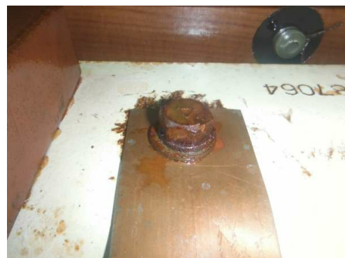
Rust formation on the ground bonding hardware on the top clamp.
