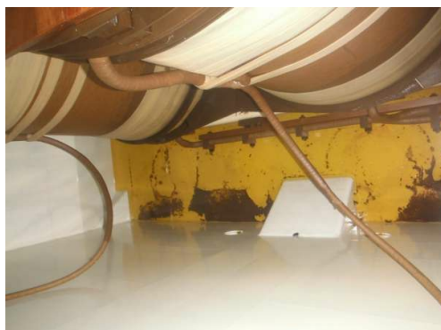
More rust deposits on the the HV side
