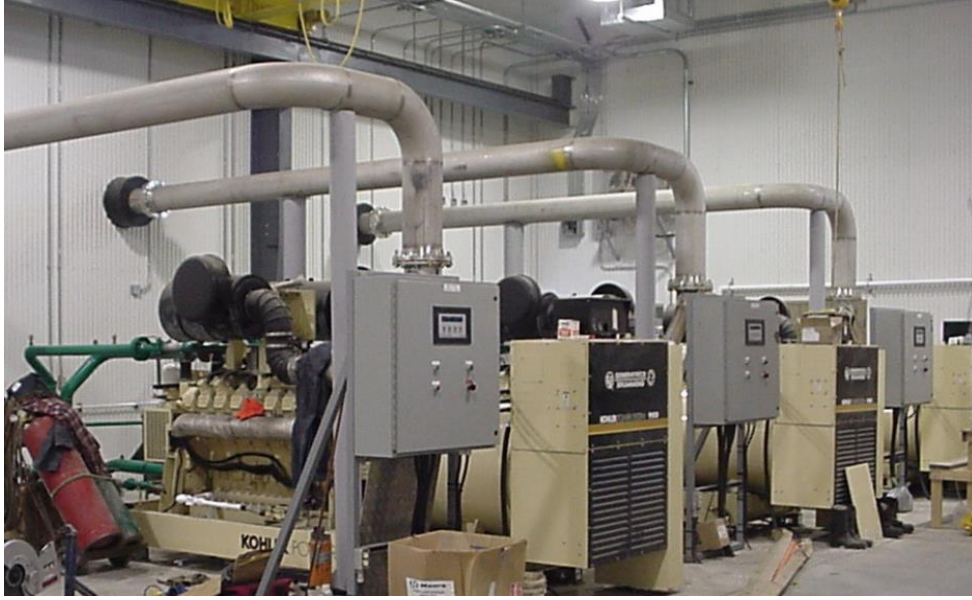
Figure 2: Nain Diesel Generators in Powerhouse
