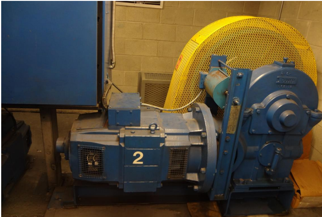
Figure 1: Hydro Place – Elevator Motor and Pulley System at the Penthouse.
