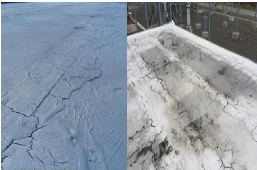
Figure 17: Terminal Station Control Buildings (Come by Chance and Sunnyside) Showing Cracking and Deterioration of the Roof Membrane System
