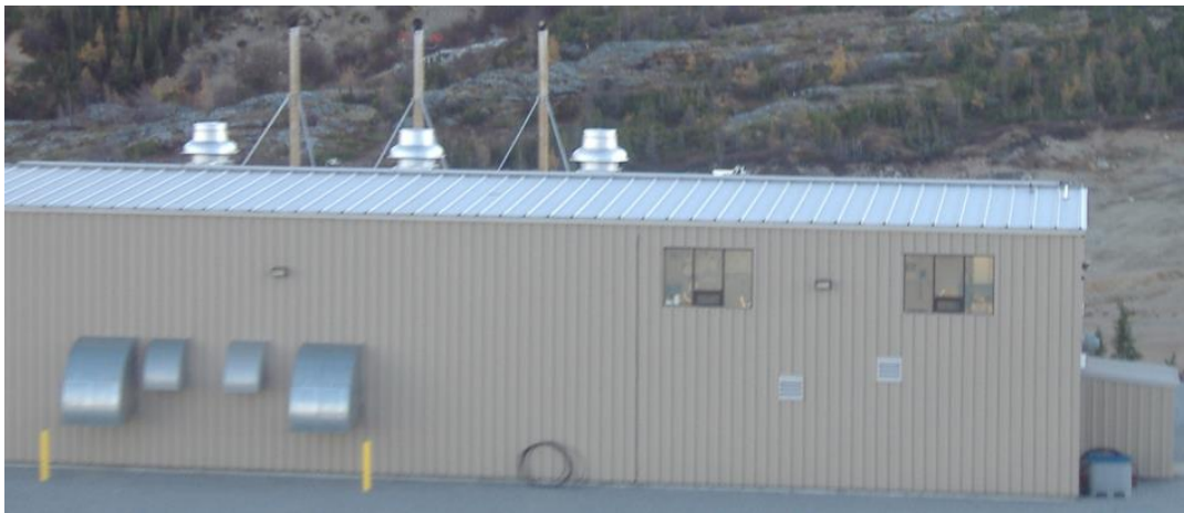
Figure 3: Nain Plant Existing Ventilation Arrangement with Roof Top Exhaust Fan
