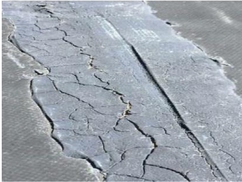
Figure 10: Roof Seam Cracking
