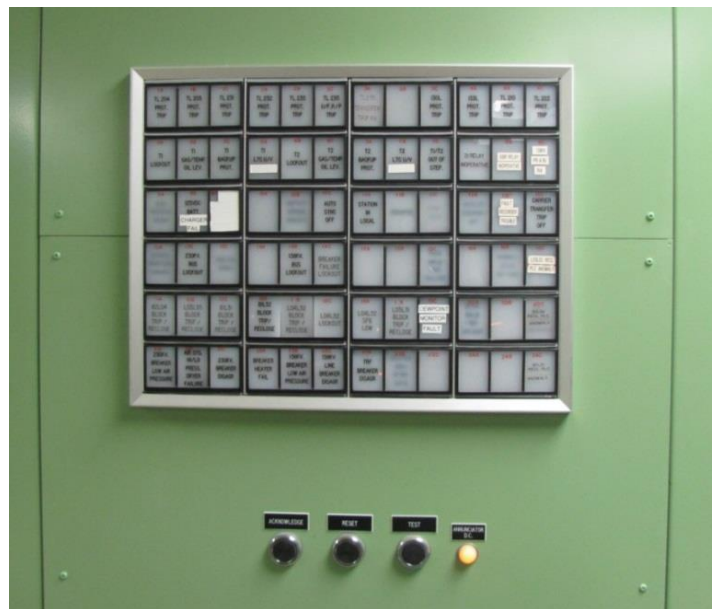
Figure 20: Annunciator Commonly Found in Hydro Terminal Stations
