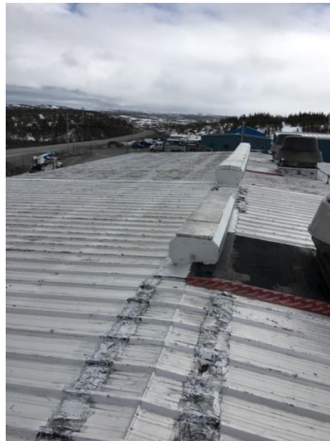
Figure 1: Typical roof panel condition
