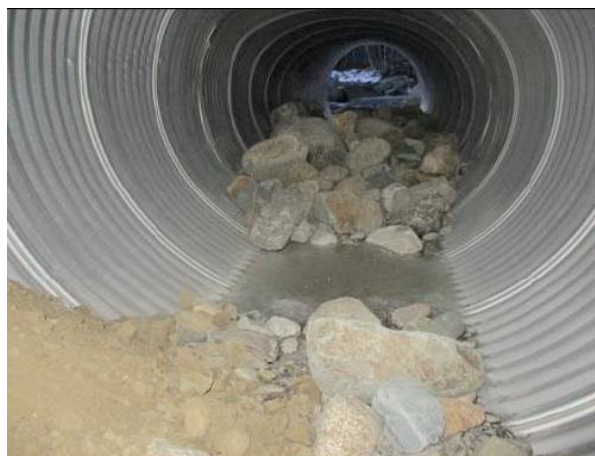
Figure 32: Bear Brook Crossing Culvert Blockage (February 2018)
