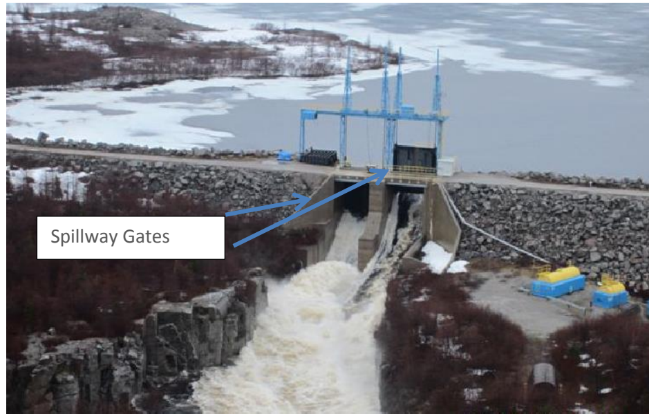
Figure 5: Burnt Dam Spillway Structure
