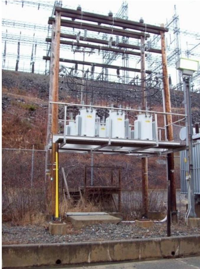
Figure 11: Bay D'Espoir– Station Service Transformers
