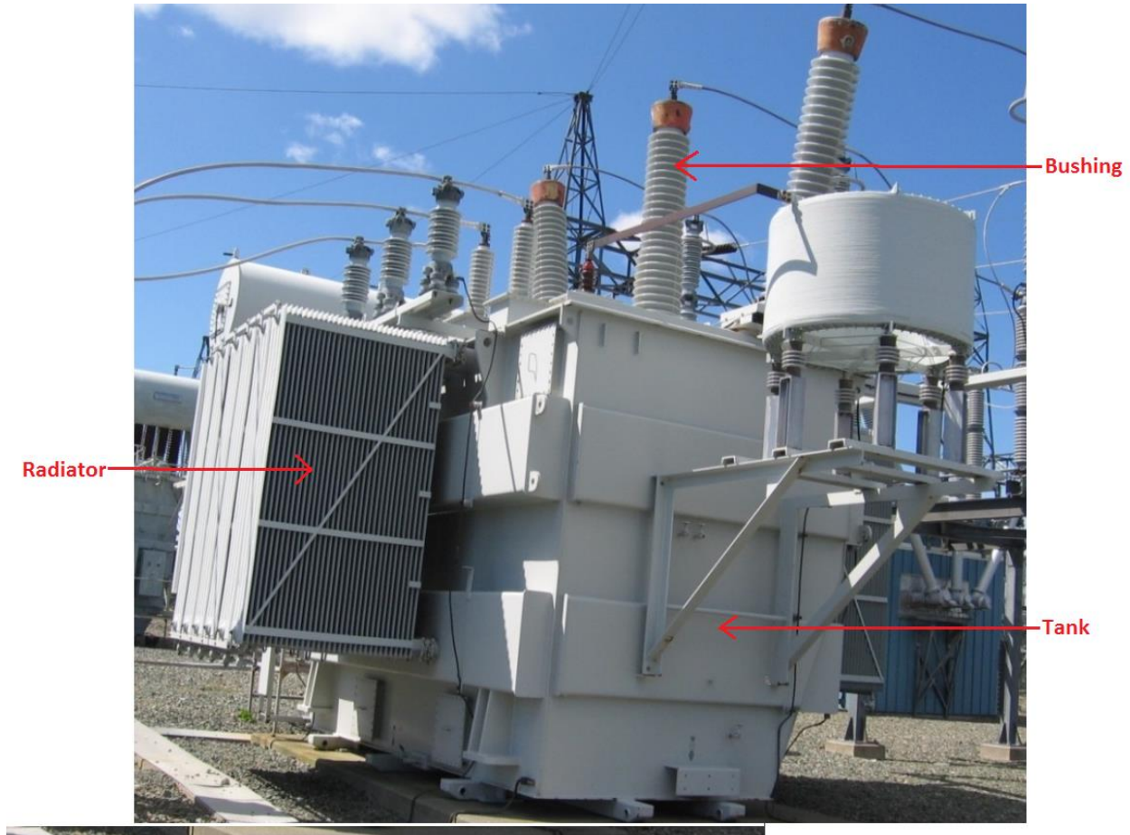
Figure 8: Power Transformer
