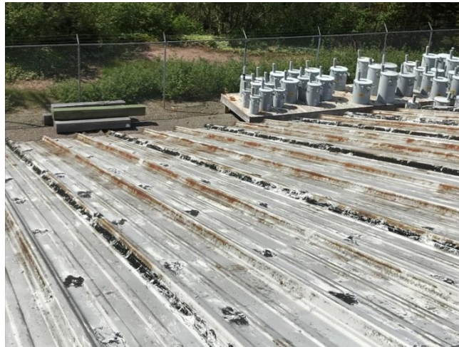
Figure 2: Previous attempt to repair leaks with elastomeric coating system
