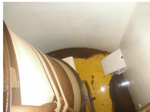
Rust deposits on the tank floor on the HV side
