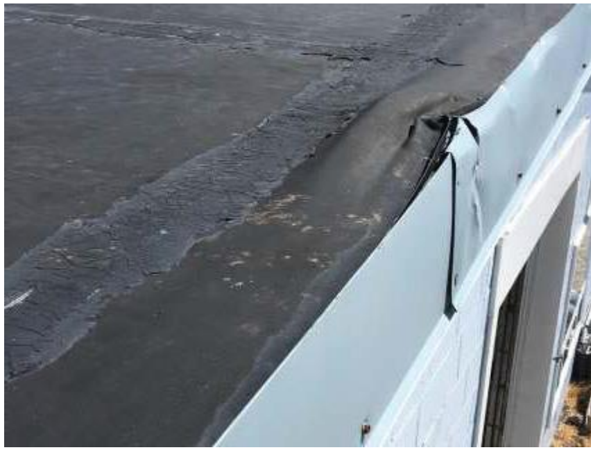
Figure 11: Roof Seams Cracking and Damage to Existing Roof
