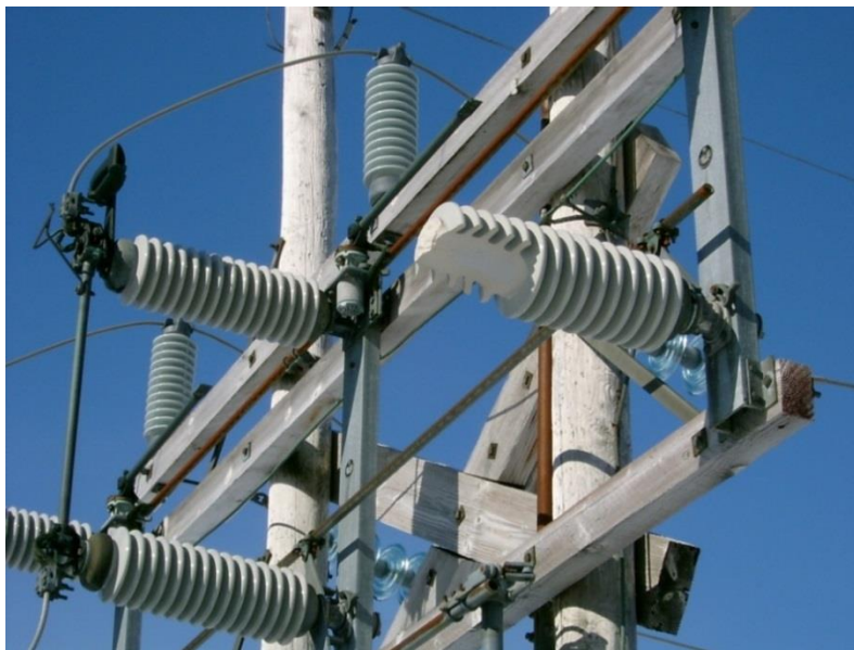
Figure 4: Broken Insulator on 69 kV Disconnect Switch
