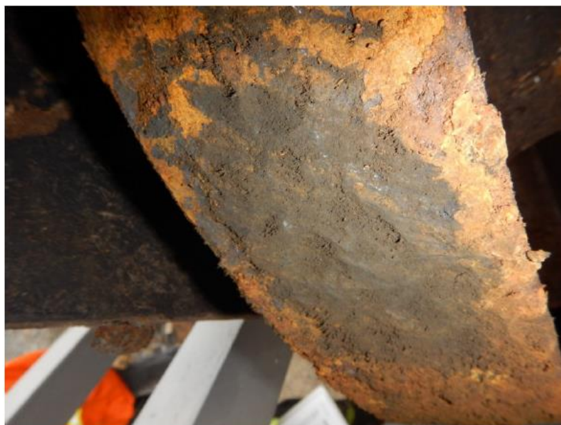
Figure 7: Pitting Corrosion on Main Rollers – Intake 1 2016
