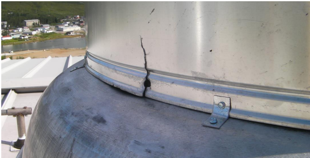
Figure 4: Nain Plant Ventilation Damaged Weather Hoods
