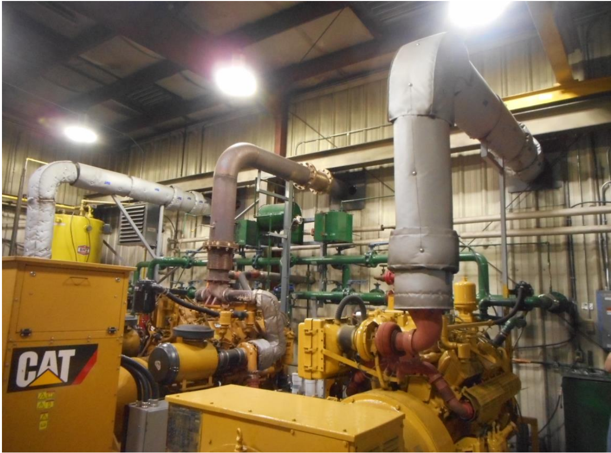
Figure 2: Diesel Generators In Powerhouse
