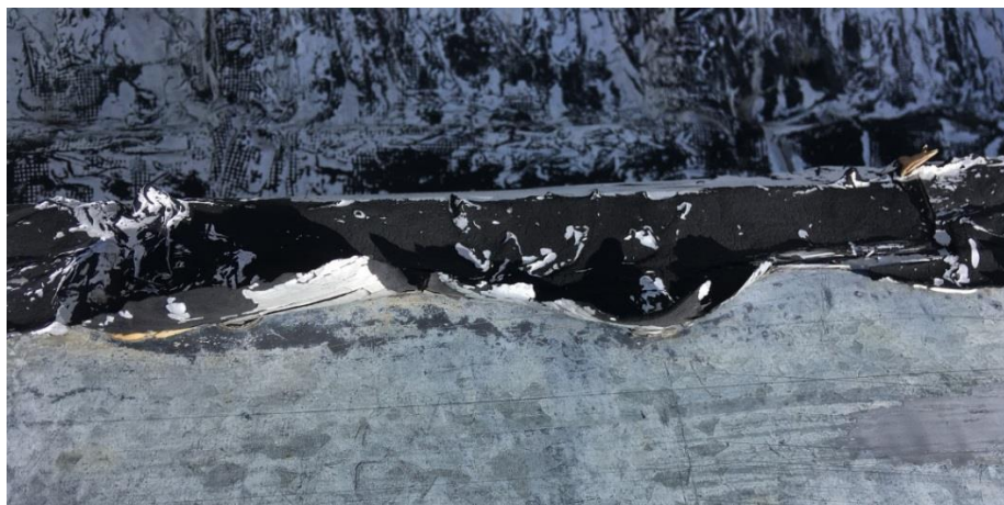
Figure 3: Ineffective elastomeric coating system
