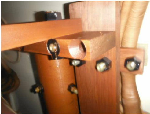
Missing bolt on the LV centre phase LV side lead structure. The bolt I found on the tank floor.
