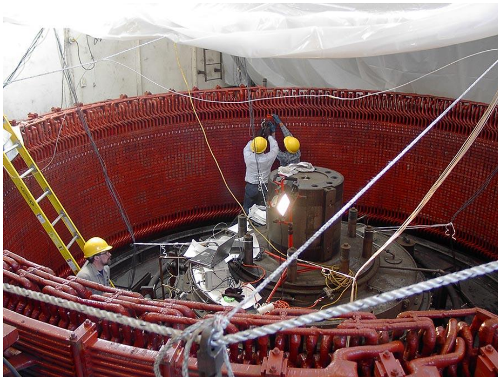
Figure 2: Stator Windings - Top View
