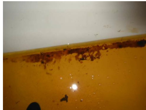
Rust deposits in the tap changer compartment.
