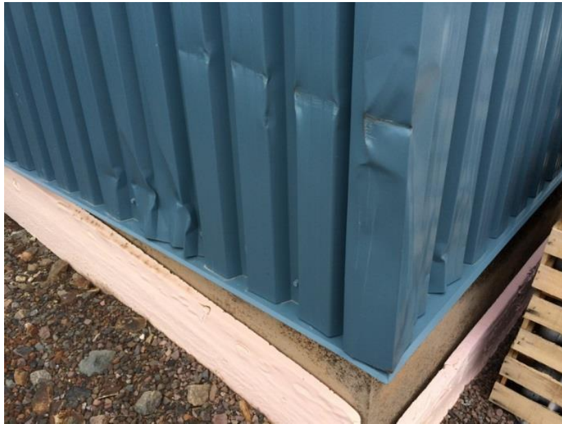
Figure 7: Damaged Siding
