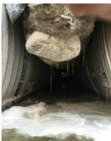
Figure 27: April 2017 - Post Weather Event - Culvert Backfill Washed Away
