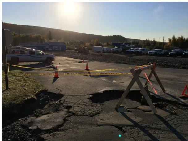
Figure 25: Post Hurricane Matthew Damage to Surrounding Infrastructure after Bear Brook Crossing Failure
