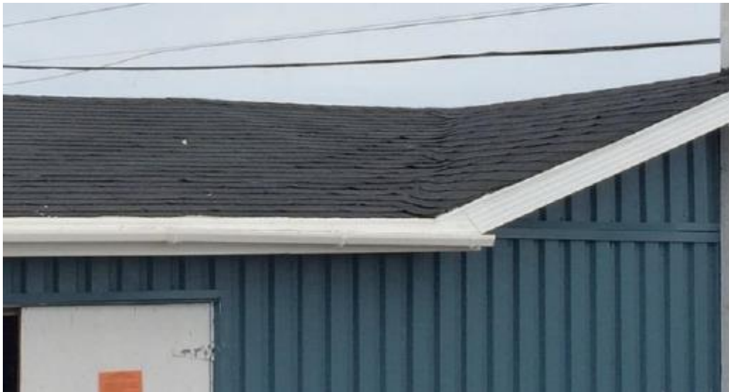
Figure 9: Deteriorated and Lifting Roof Shingles
