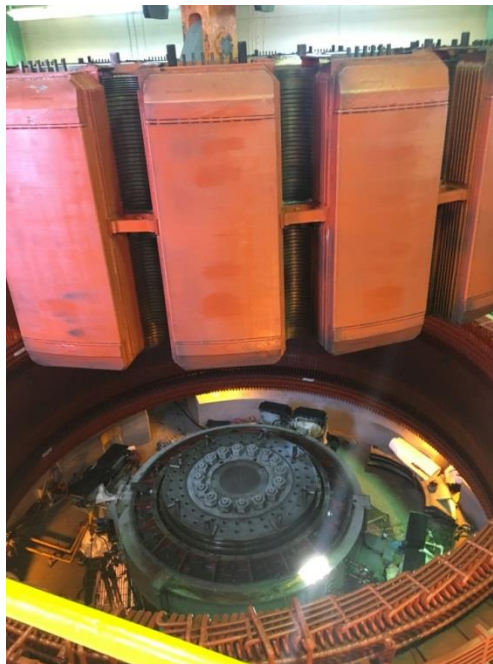
Figure 3: Dismantled Generator
